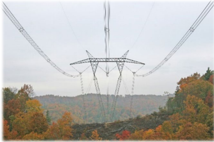
765kV Single-circuit (6-conductor)
