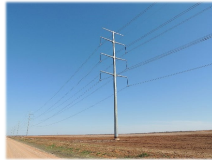
345kV Traditional Double-circuit (3-conductor)
