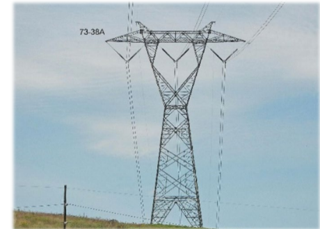
500kV Single-circuit (3-conductor)
